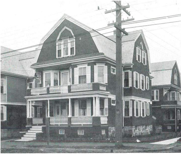
Bay State Avenue, ca. 1899. A real estate promotion featured this photograph of Bay State Avenue shortly after the first houses were built by H. D. McGray. Decorative oriels and millwork enhanced the shingle covered, gambrel-roofed designs.
