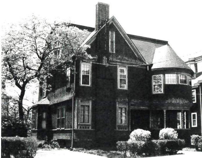
152 Summer Street, 1895. George F. Loring, architect. Smooth, shingle-clad wall surfaces, simple ornamentation, and circular turrets and verandas integrated into the overall design are characteristics of the Shingle Style, which appeared in Somerville in the 1890s.
