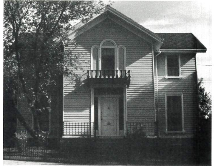
Charles Williams House, 108 Cross, ca. 1848. One of the best conserved early Italianate houses in Somerville. The Palladian window motif and glazed transom and sidelights of the projecting pavilion are features of the original design. Williams was a Boston hat dealer.
