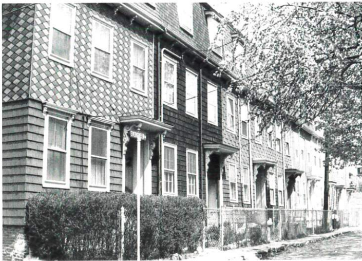
Evergreen Terrace, off Porter Street. ca. 1873. By 1870, Milk Row, now Somerville Avenue, had several large factories, such as the Middlesex Bleachery, which employed local workers. This eight-unit, mansard-roofed row is one of many built after the Civil War to house Somerville's growing number of factory workers.
