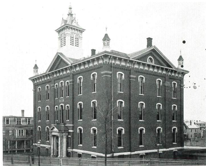
Luther V. Bell School. Vinal Avenue, 1874. Shephard S. Woodcock, architect(?). Razed.
