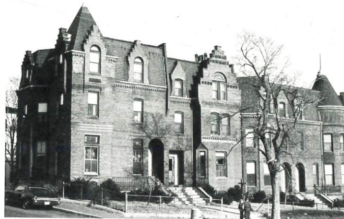
Langmaid Terrace, 359-365 Broadway, 1889. Rowhouses and apartment rows began to replace large single family houses on Winter Hill in the 1880s and 1890s. Among the finest apartment row in the city is this brick and terra cotta building, with a variety of roofs and crenellated parapets. Of note is the stained glass work and terra cotta inset "Langmaid Terrace" in the front parapet.
