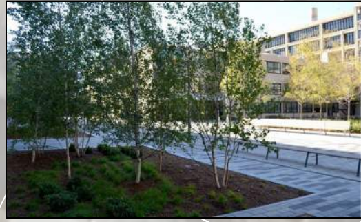
Precedent Image - MIT Campus Bioretention landscape retains stormwater subgrade, instead of ponding at the surface; landscape grade is even with surrounding area
