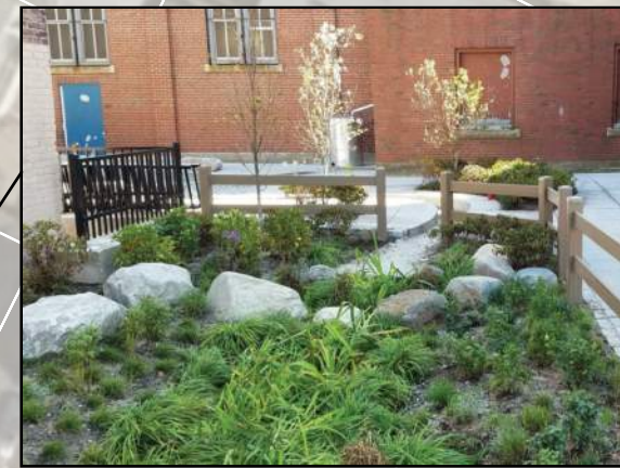
Precedent Image - Hernandez Elementary School Roxbury Stormwater routed to interactive bioretention landscape
