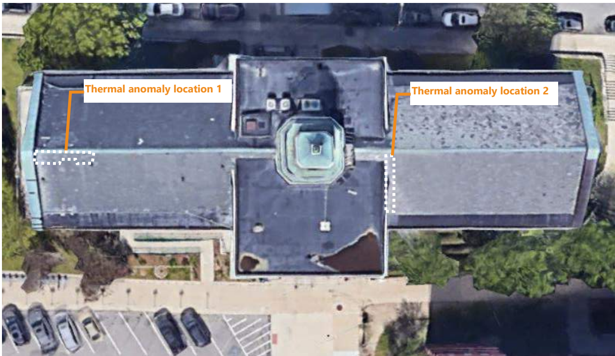
Figure 12. Thermal anomaly locations at City Hall.
