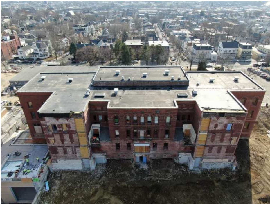
Figure 3. 81 Highland Avenue (High School)
