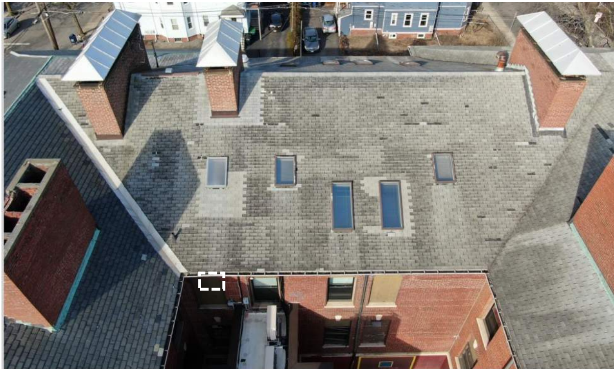
Figure 17. Overall view of the Brown School (central portion)
