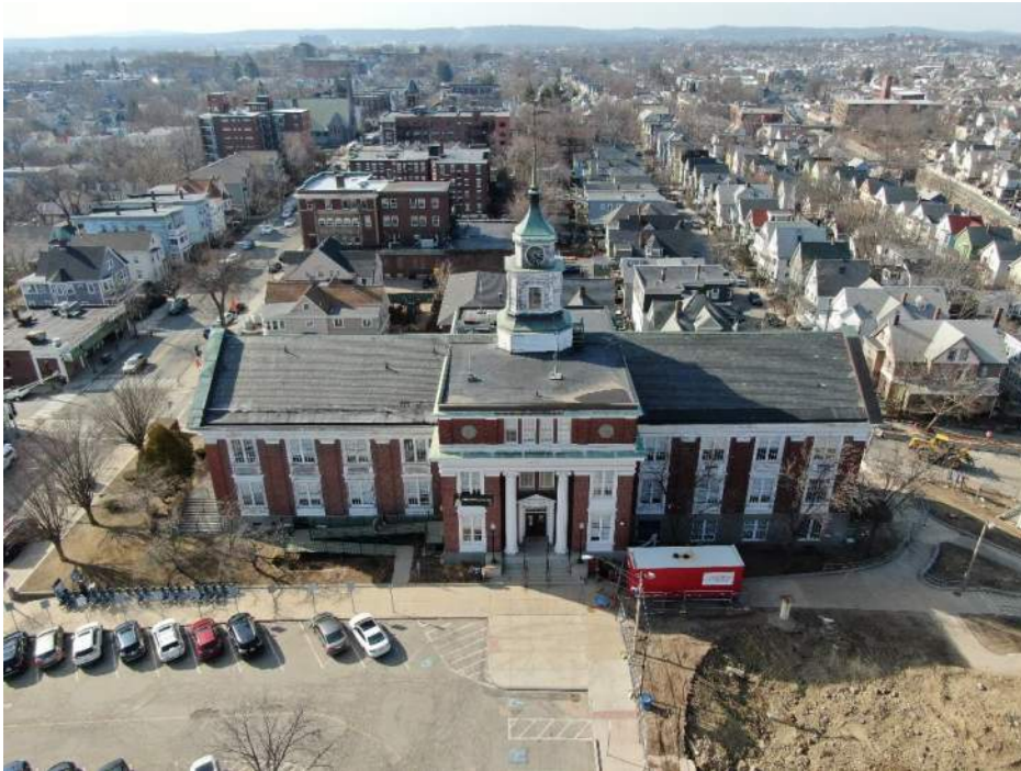
Figure 2. 93 Highland Avenue (City Hall)
