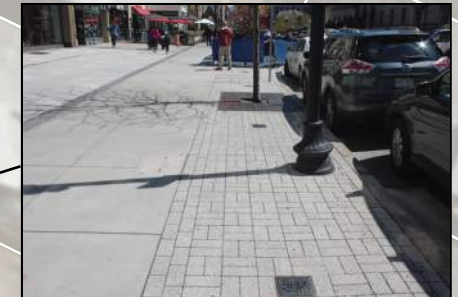
Precedent Image - City of Boston Conventional concrete sidewalk pitches to permeable paver strip with underdrains
