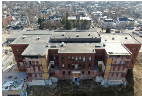
Existing photos of the south (top) and north facades
