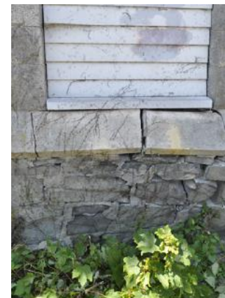
Cracked water table and random ashlar base displacement and loss of pointing; loading dock and garage door at center window, east elevation
