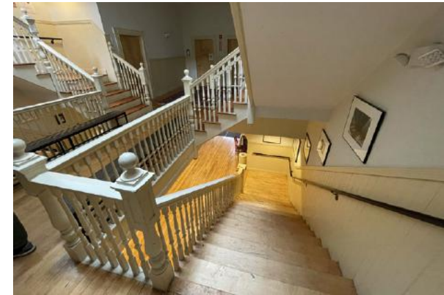
Second Floor Landing, Main Stair
