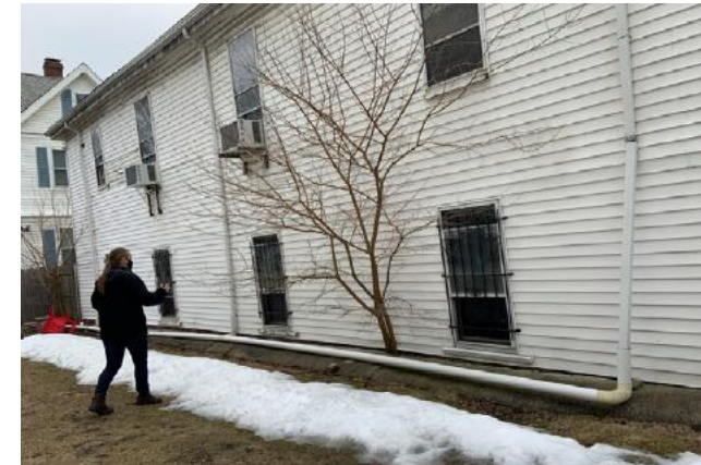
External downspout drainage at the north elevation
