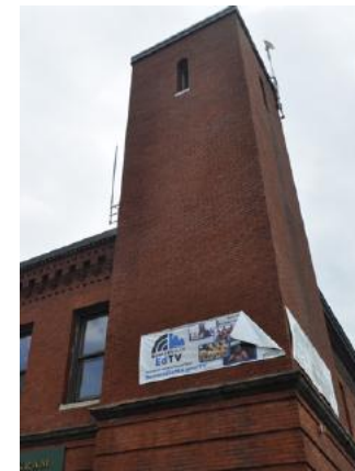
Corner tower with soiling pattern evident; graffiti paint-over, northwest corner
