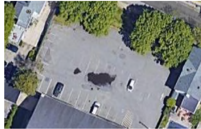
Google Earth aerial of ponding occurring in parking lot
