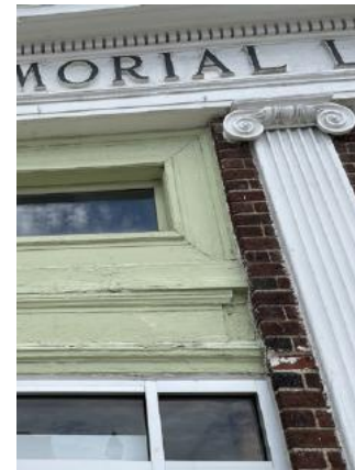
Weathering of exterior millwork; original half-pilaster detail
