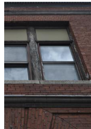
Lost roof shingles at one-story roof; weathered window millwork
