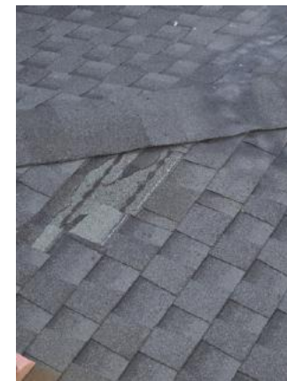
Lost roof shingles at one-story roof; weathered window millwork
