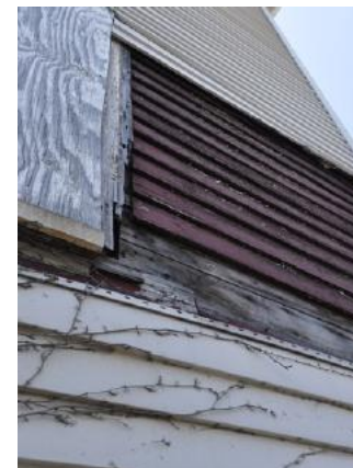
Wood clapboard siding beneath aluminum at west wing; brick displacement
