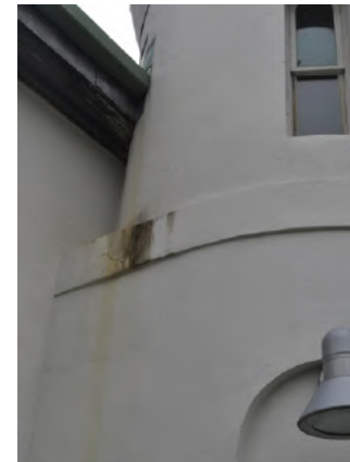
Damaged soffit and runoff staining; delamination of paint coating on stucco
