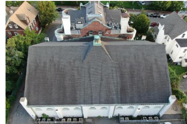
Drone photograph of Armory roof
