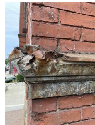
Damage to galvanized metal cornice at southeast corner of building; spalling and damage at entry brick return
