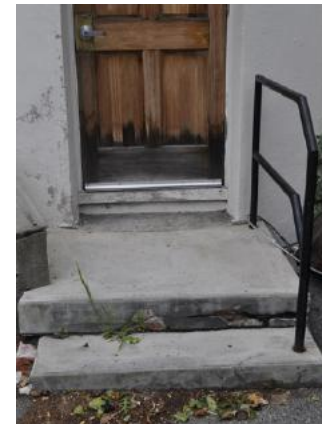
Stoop and egress door deterioration; window grate deterioration
