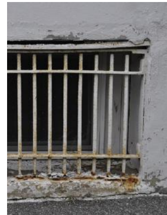
Stoop and egress door deterioration; window grate deterioration
