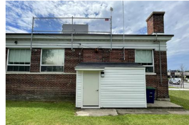
Rear addition over basement stair with second exit
