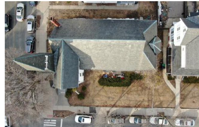
Drone photograph of church roof
