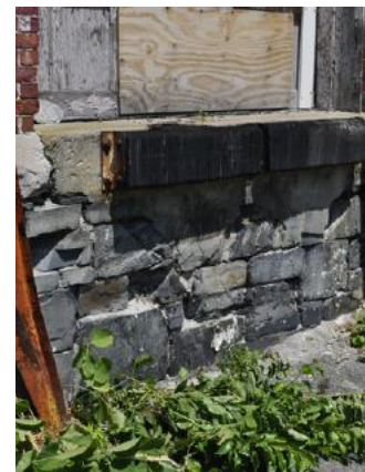
Cracked water table and random ashlar base displacement and loss of pointing; loading dock and garage door at center window, east elevation
