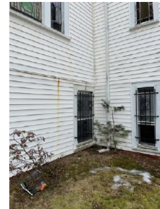
External downspout to planted area
