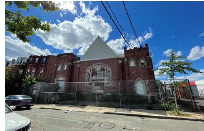
Street facade, looking west
