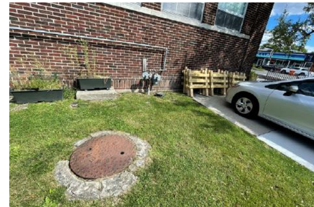
Sewer manhole west of building
