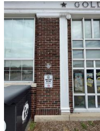
Weathering of exterior millwork; original half-pilaster detail
