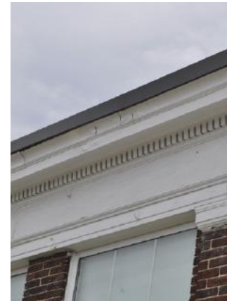
Deteriorated paint at the cornice; unsympathetic brick infill at window
