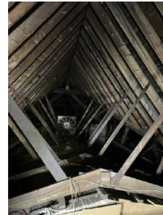
Main attic roof trusses; typical brick cracking and displacement on buttress
