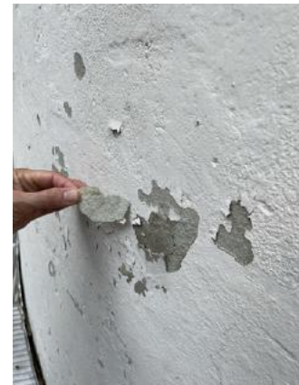
Damaged soffit and runoff staining; delamination of paint coating on stucco
