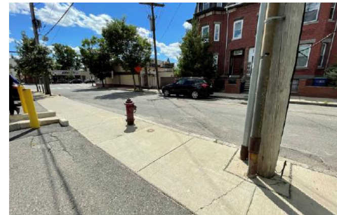
Condition of hardscape and sidewalk, Cross Street East
