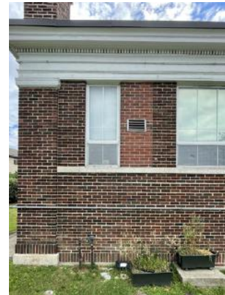
Deteriorated paint at the cornice; unsympathetic brick infill at window
