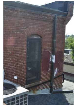
Corner tower with soiling pattern evident; graffiti paint-over, northwest corner
