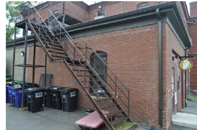
External steel fire escape, north elevation
