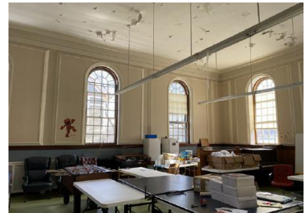
Main Courtroom, looking southeast
