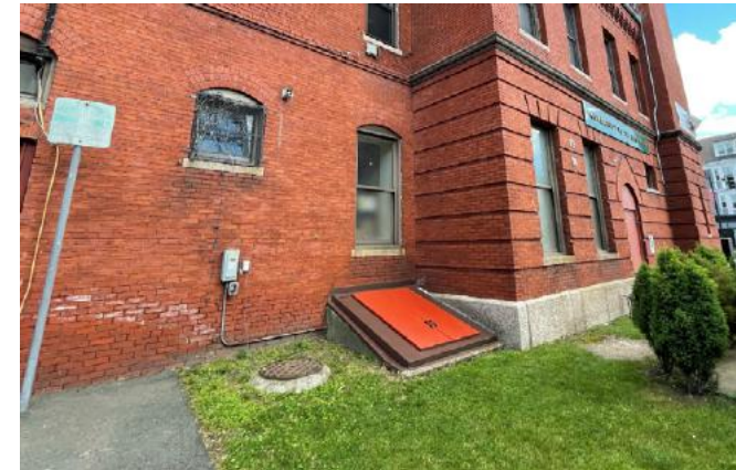
West side of building: manhole and basement access hatch
