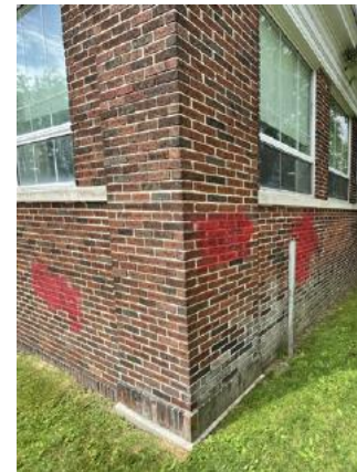
Graffiti paint-over and efflorescence; Broadway Plaza seating
