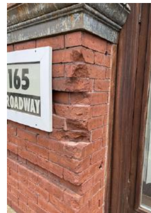
Damage to galvanized metal cornice at southeast corner of building; spalling and damage at entry brick return
