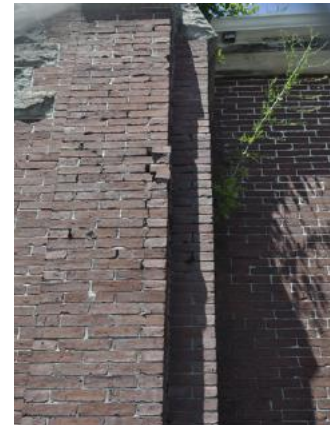
Main attic roof trusses; typical brick cracking and displacement on buttress
