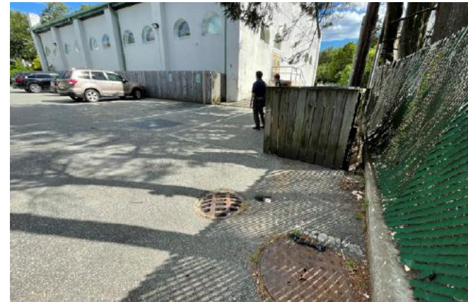
Catch basin and sewer manhole at west end of parking lot
