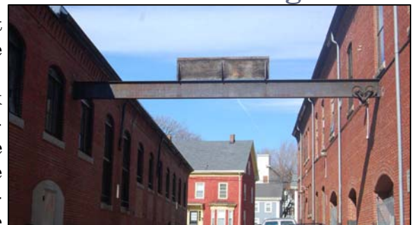
440 Somerville Avenue, metal hoist
