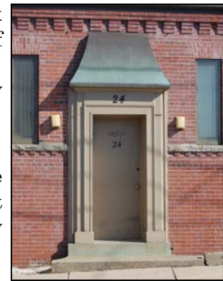
24 Dane Street, Boiler House copper canopy
