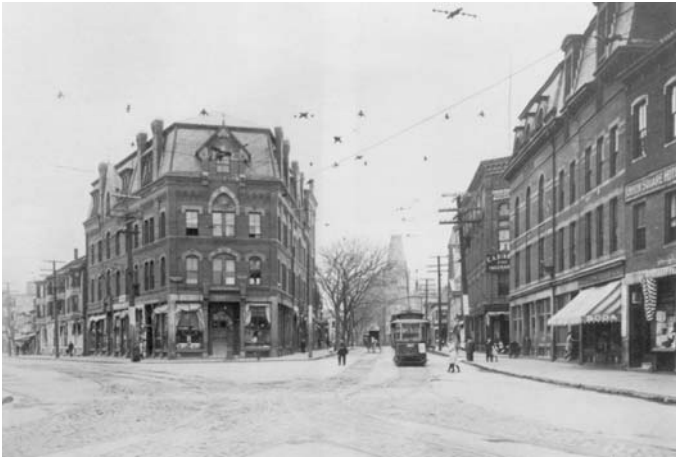
Hill Building at the junction of Bow Street and Somerville Avenue – 1915
