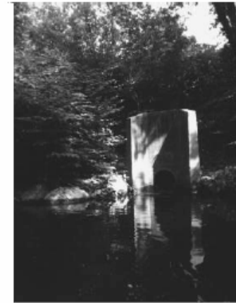
Somerville storm drains
