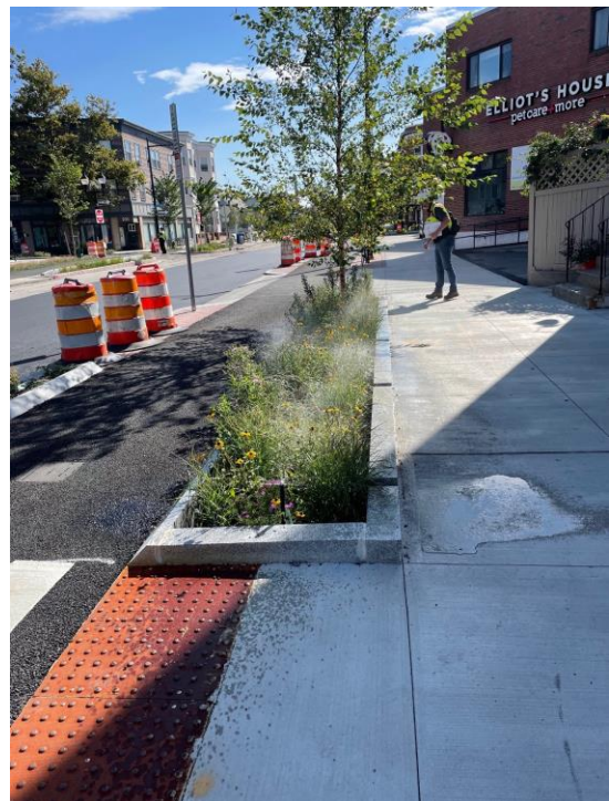
One of the planters installed as part of the SAUSI project.
