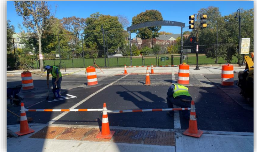
Raised crosswalk construction, October 2022
