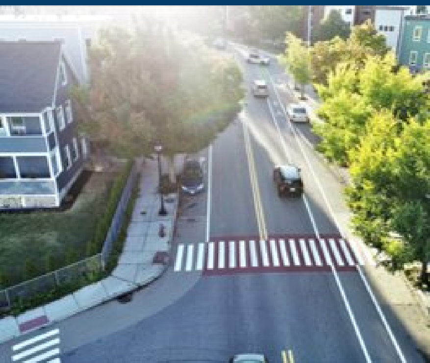
Red-backed crosswalks painted as a quick and proven way to slow vehicles at crossings
