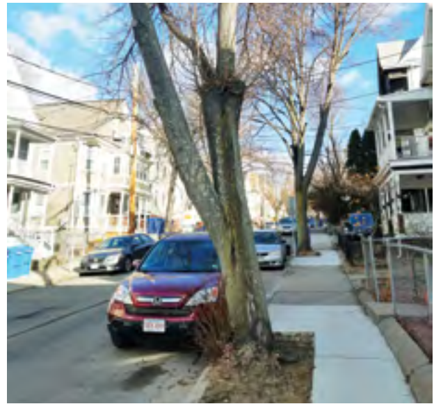
Note the color changes of the sidewalk. The lighter gray color of the sidewalk is where the sidewalk has been replaced.
