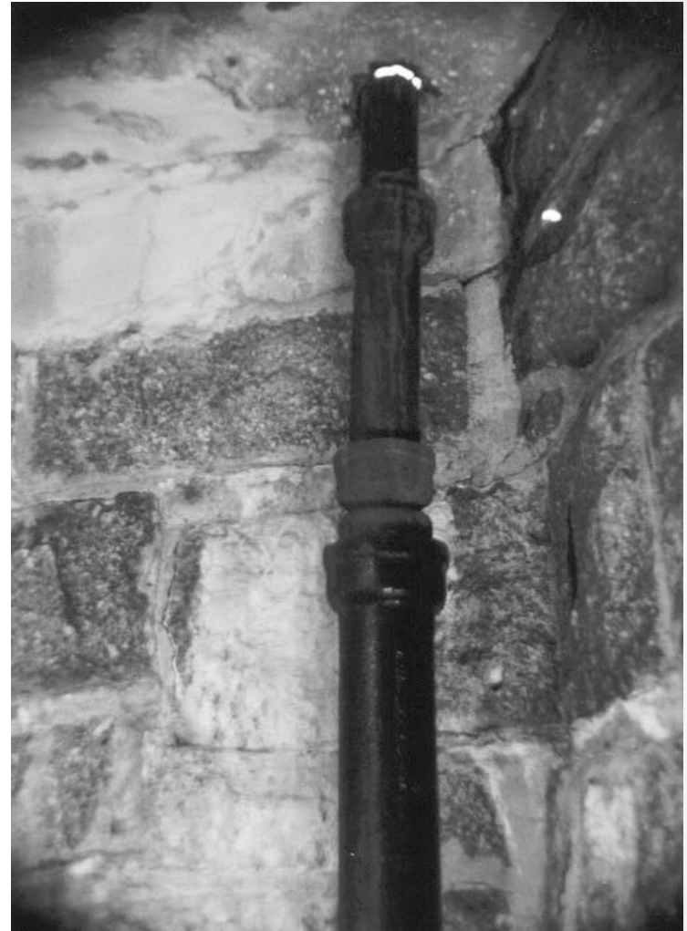
Drainpipe disconnected
