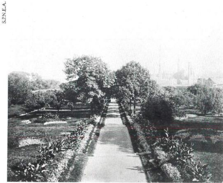
McLean Asylum Terrace and Walk with View of North Packing Plant. Photo ca. 1885. This photograph well explains the conflicting land use of the Cobble Hill area. At right is the North Packing Plant complex, which was one of the city's largest and most odiferous slaughterhouses.
