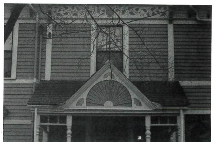
2 Bigelow Street, photograph 1989. A screened-in porch was removed to better display the sunburst design over the entrance portico. The stick work which articulates the structural design has been enhanced by a contrasting color scheme. Even the chain link fence was replaced with a more appropriate wrought iron fence and the original brick sidewalks were retained.
