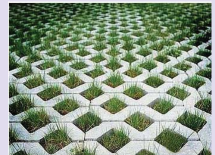
Pervious pavers use materials that allow water to percolate through.
