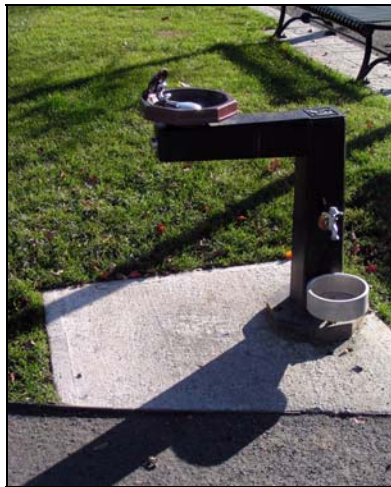
Perry Park (2007) Water fountain has hand-operated push button with clear access and adequate knee space.
