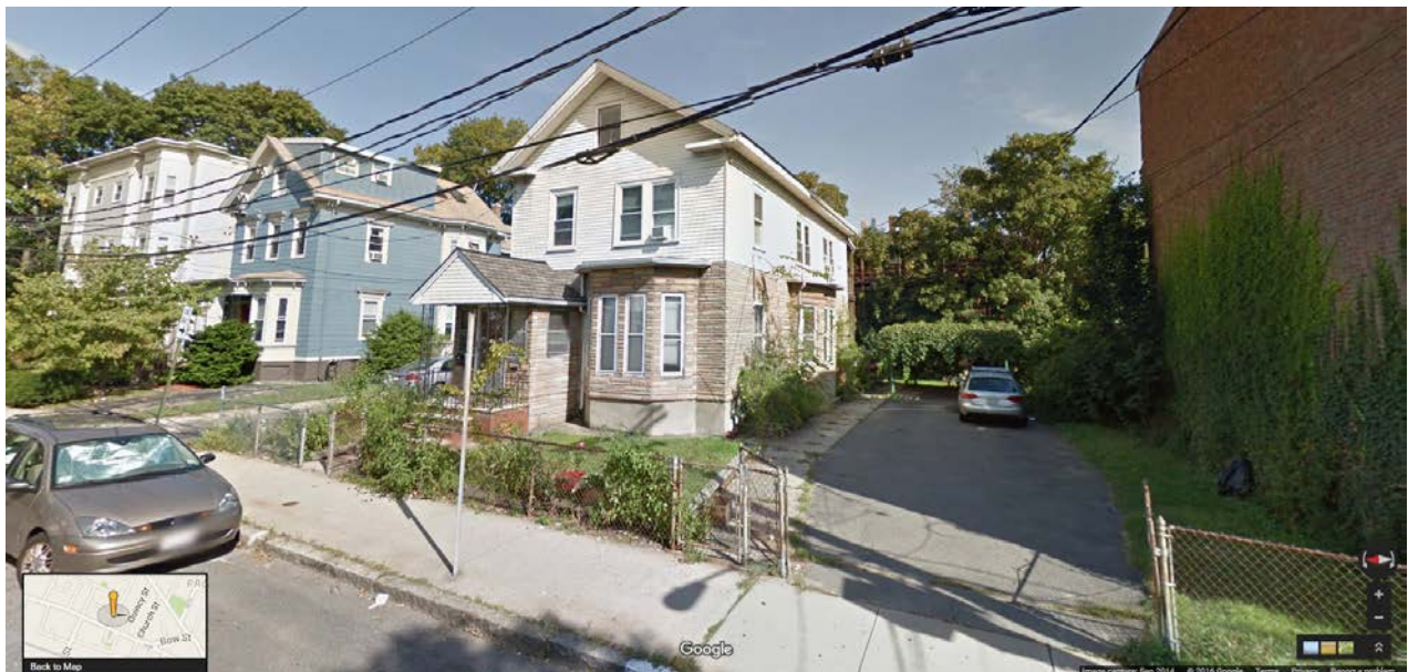
Street view of structure
