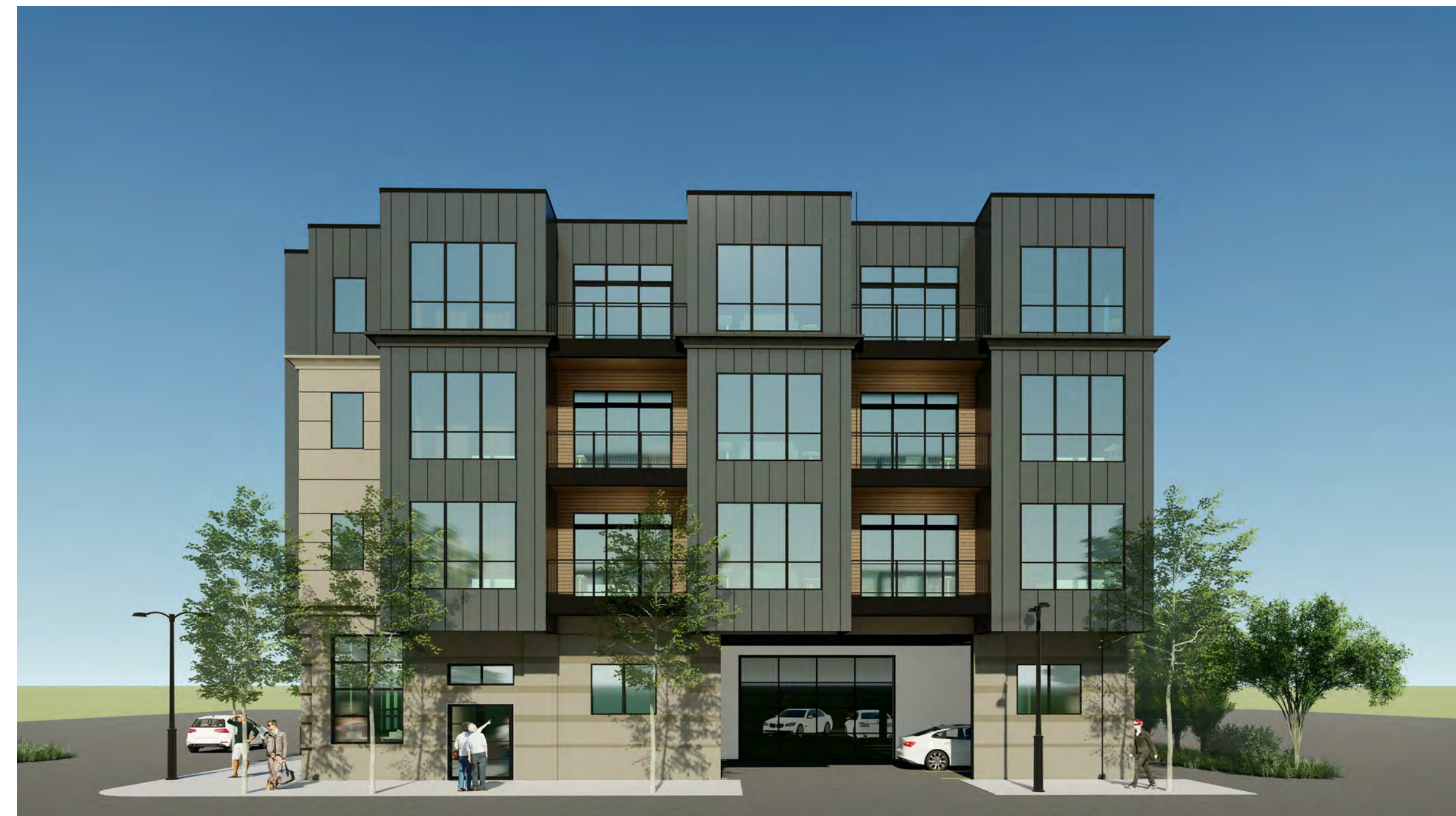
BEDFORD STREET ELEVATION
