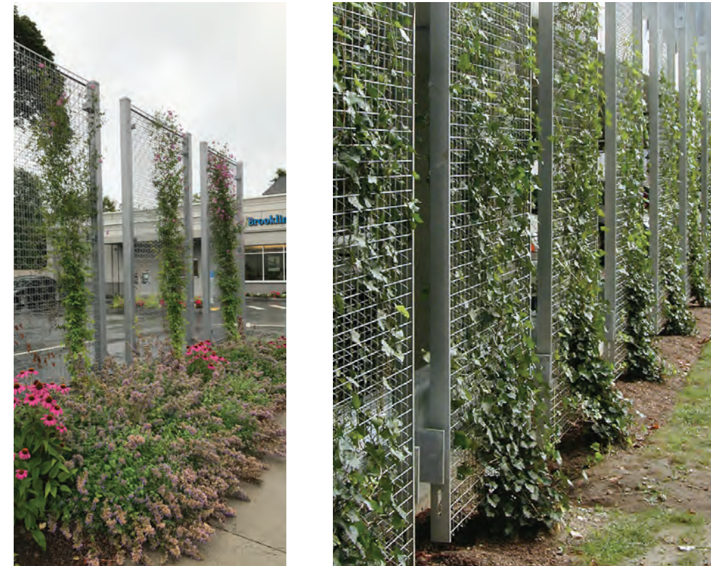
greenscreen with vines to screen drop off
