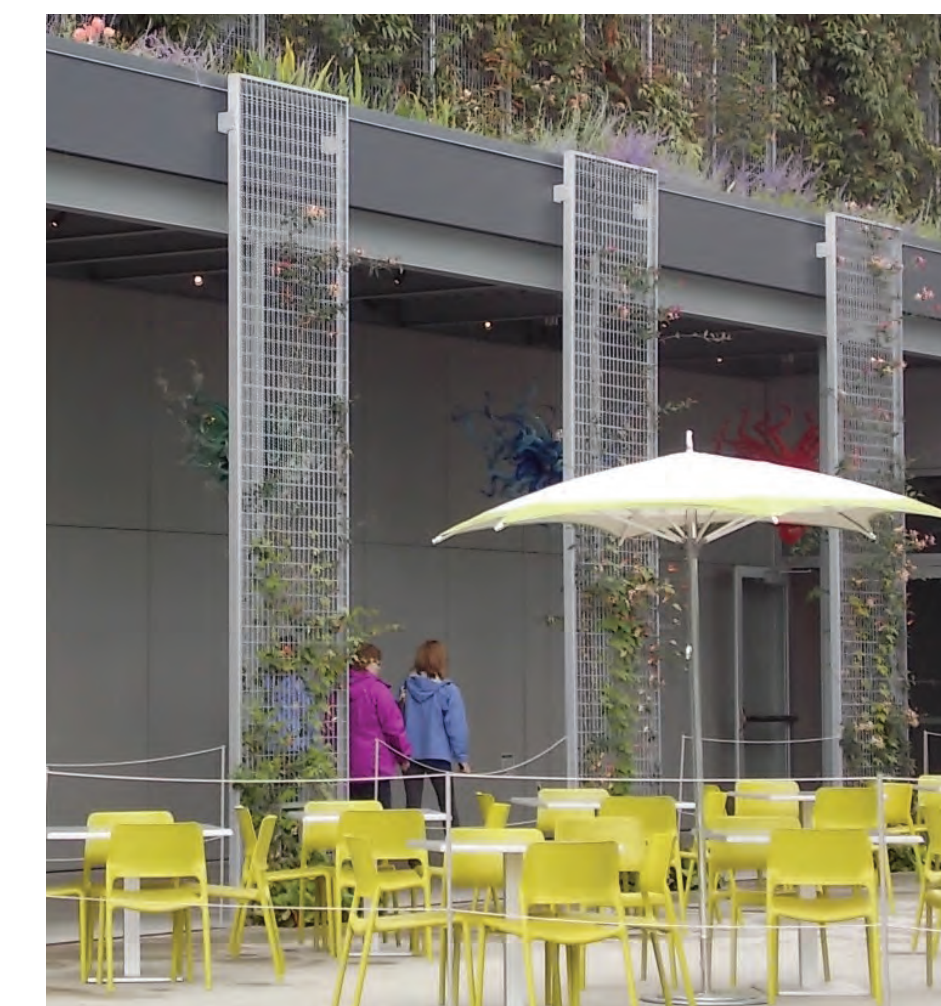
greenscreens along adjacent building face
