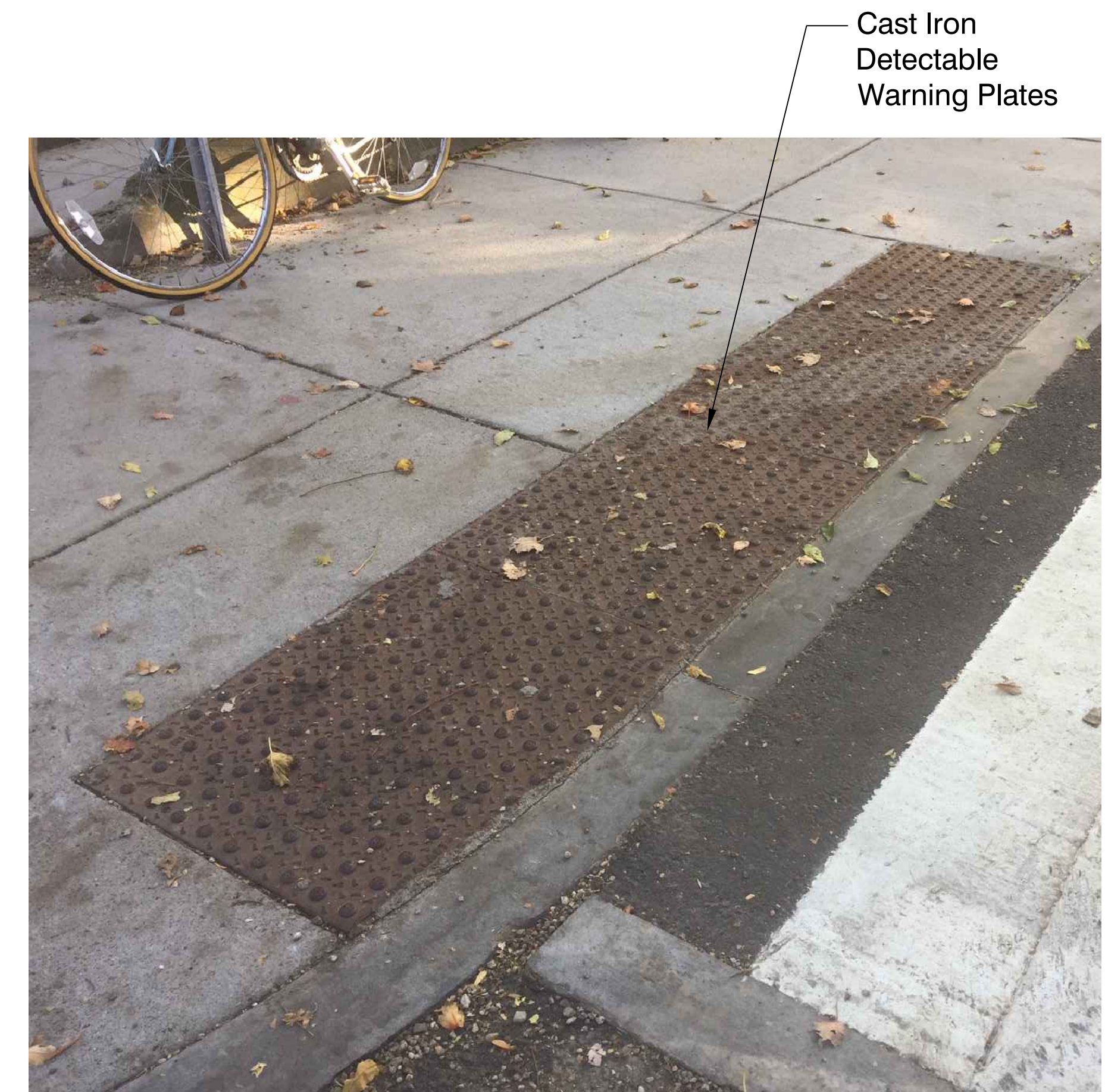
5 Detectable Warning Strip Scale: NTS Detail
