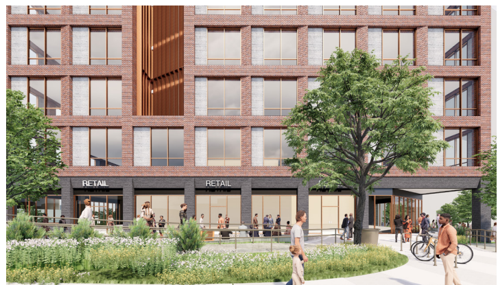
West Facade Retail Facing Civic Plaza Presented
