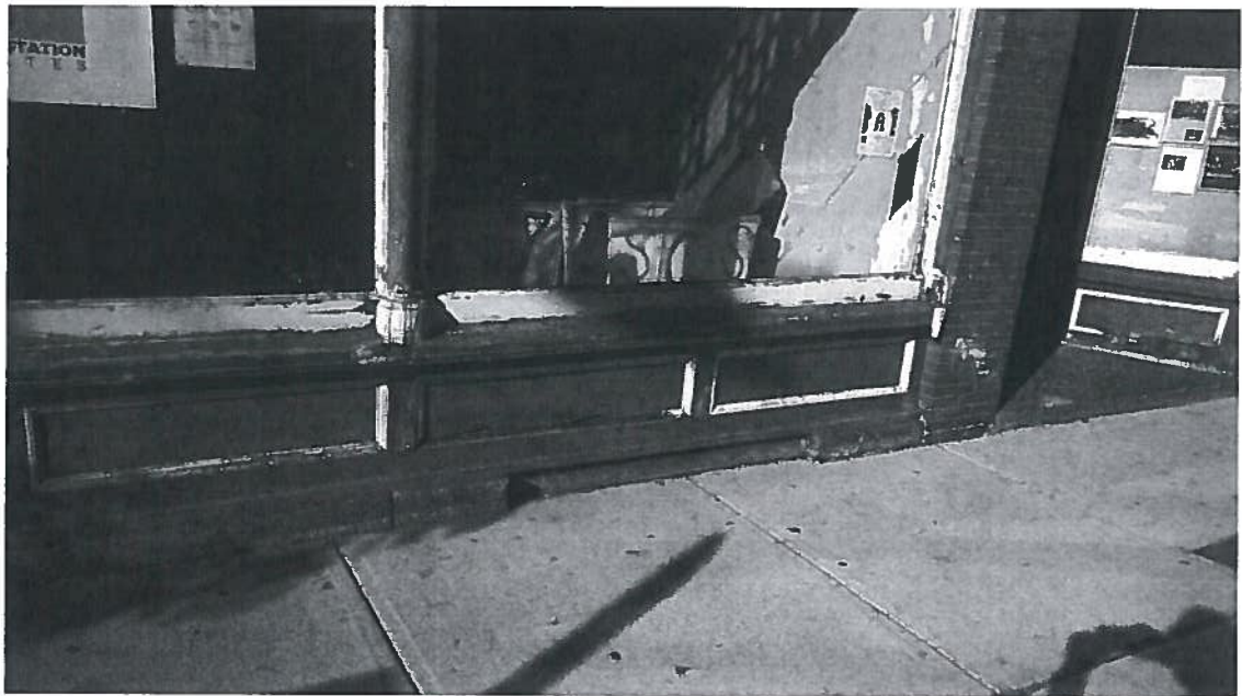
Plywood-Sheathed and Wood-Stud Base, Sill, Center and End Decorative Wood Posts, and Brick Column at Lower Glazing of Storefront Construction
