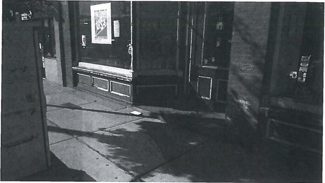
Lower Storefront at Entry to 31 Union Square
