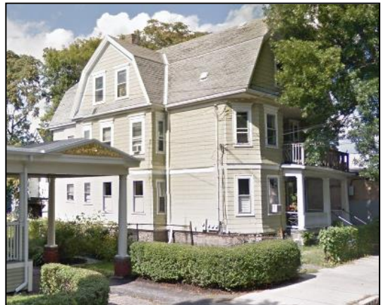
View from Willow Avenue prior to the siding being removed.
