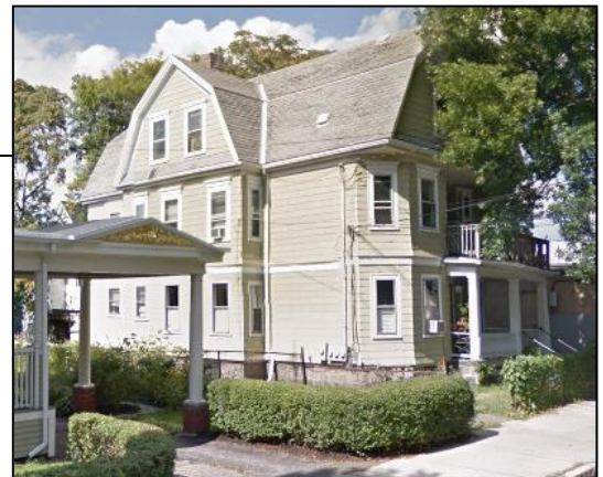
View from Willow Avenue prior to the siding being removed.
