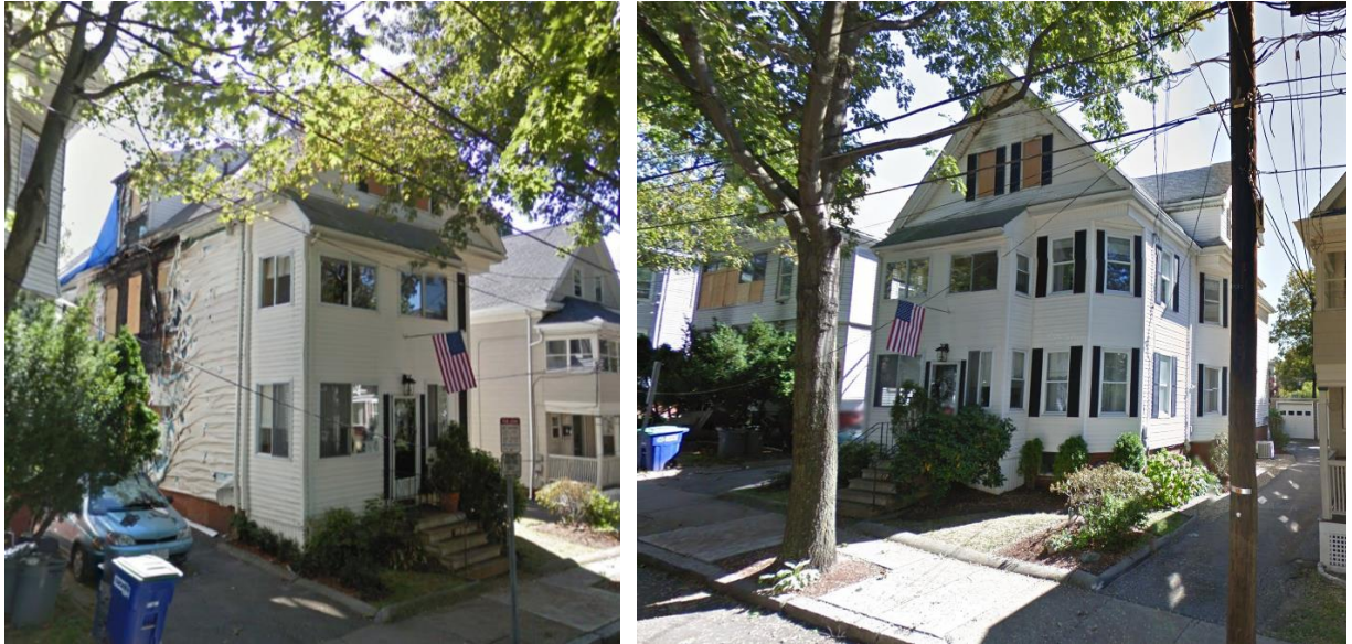
Views of 17 Banks Street after the fire.
