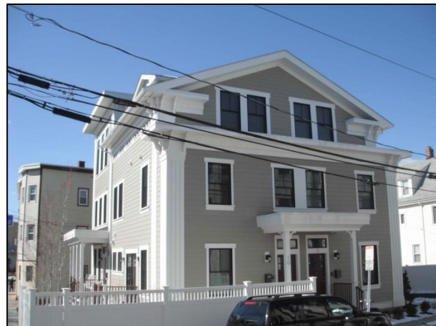
Unit #3 is at the rear of the above building. This property sits at the corner of Beech and Pitman Streets.
