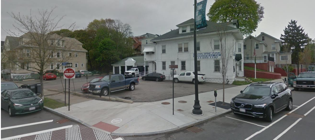
View of the locus from the intersection of Broadway and Pennsylvania Avenue.
