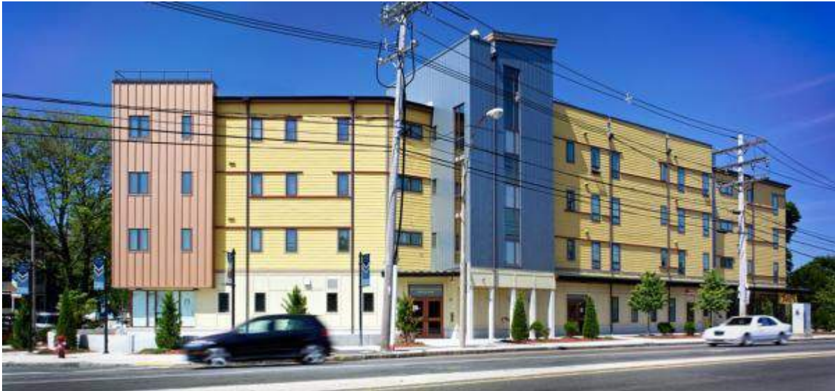
Somerville Community Corp. – St. Polycarp Village
