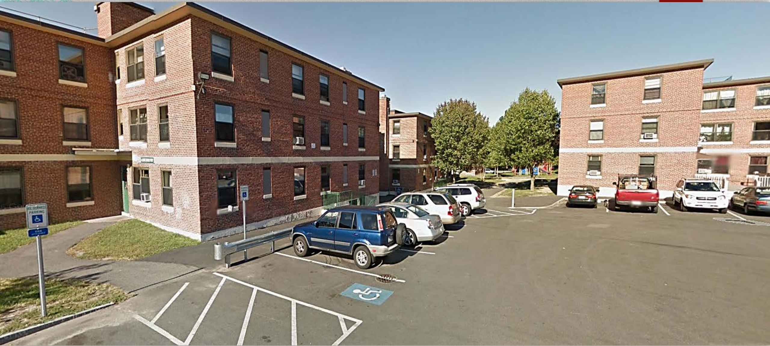
VIEW FROM INTERIOR PARKING LOT OF CLARENDON
