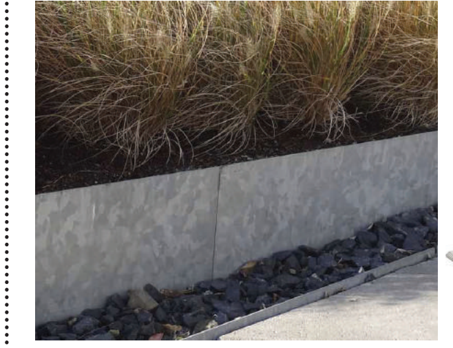
Metal Curb at Tall Plant Bed
