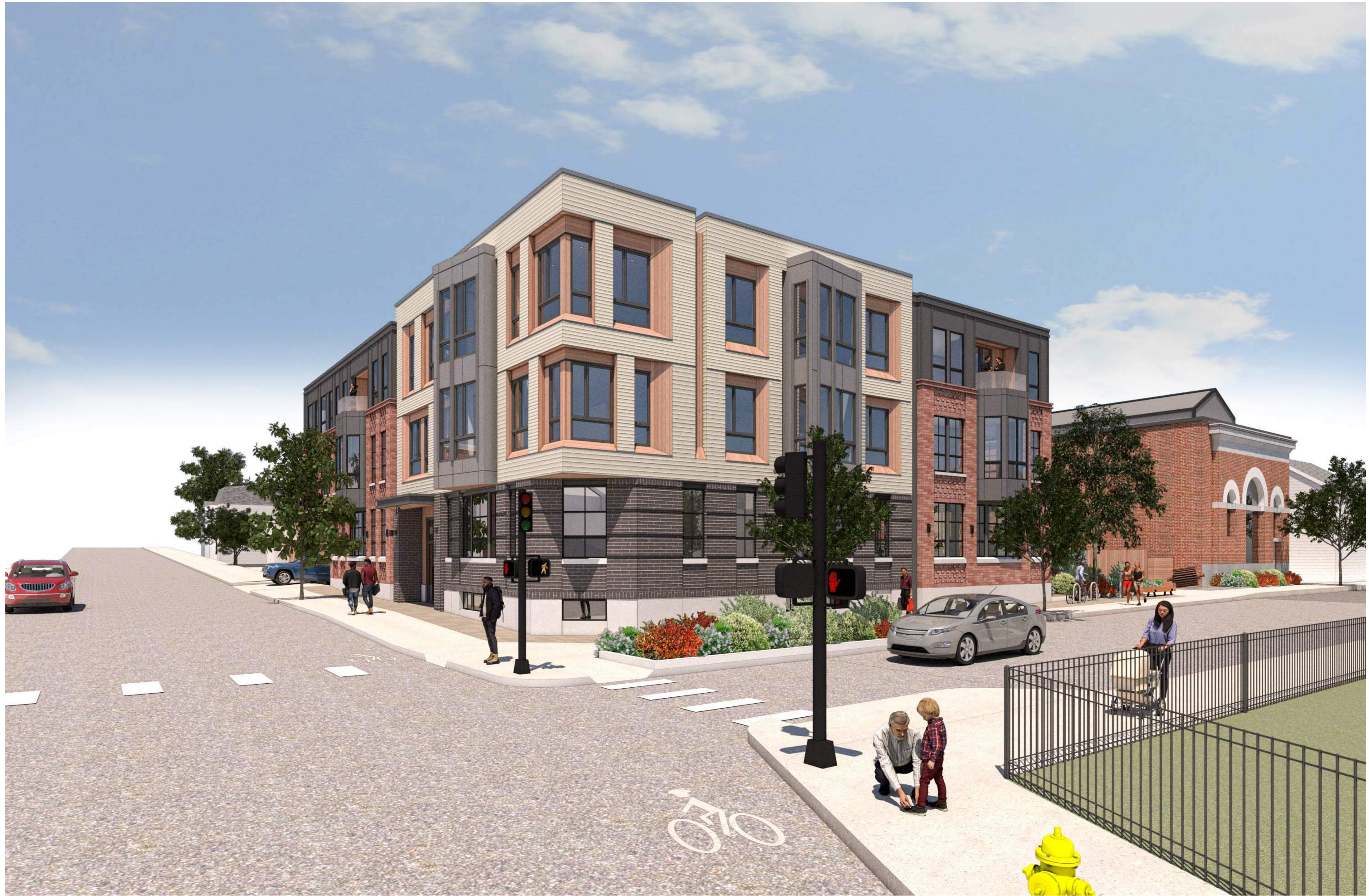
1 VIEW OF BUILDING FROM CORNER OF SCHOOL AND SUMMER STREET
