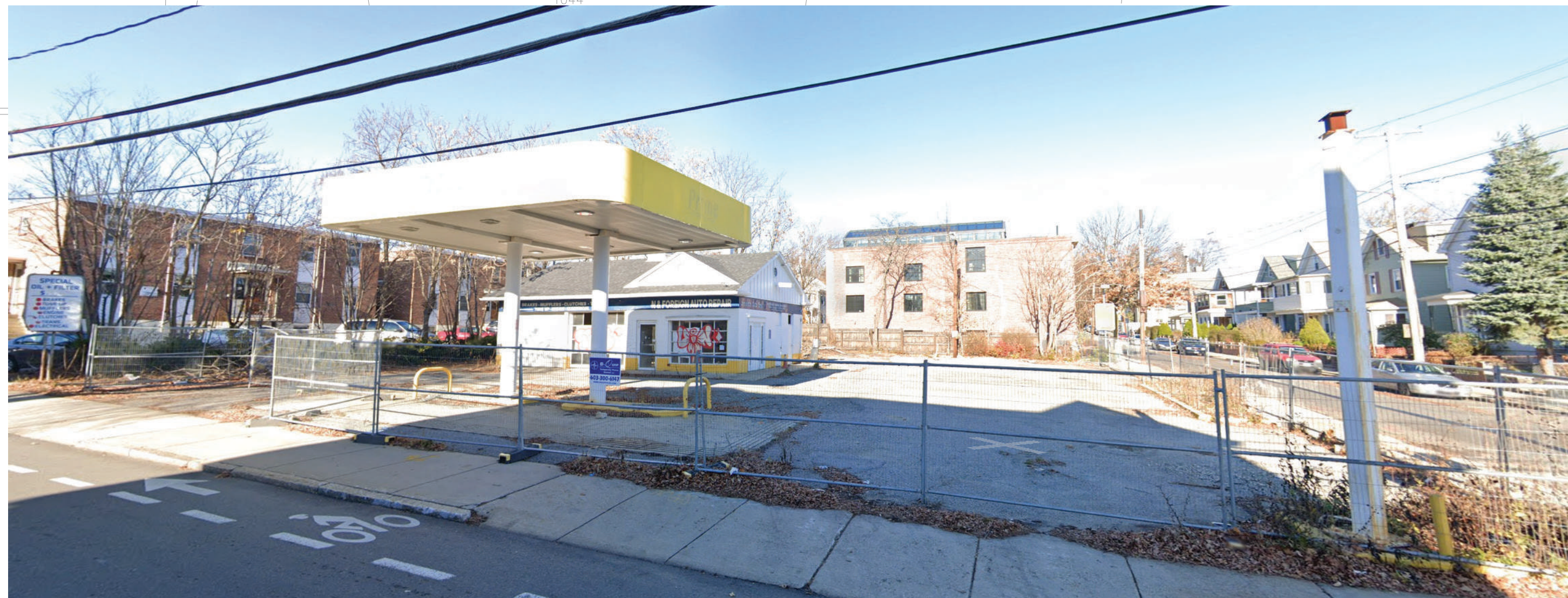
EXISTING CONDITIONS FROM SUMMER STREET
