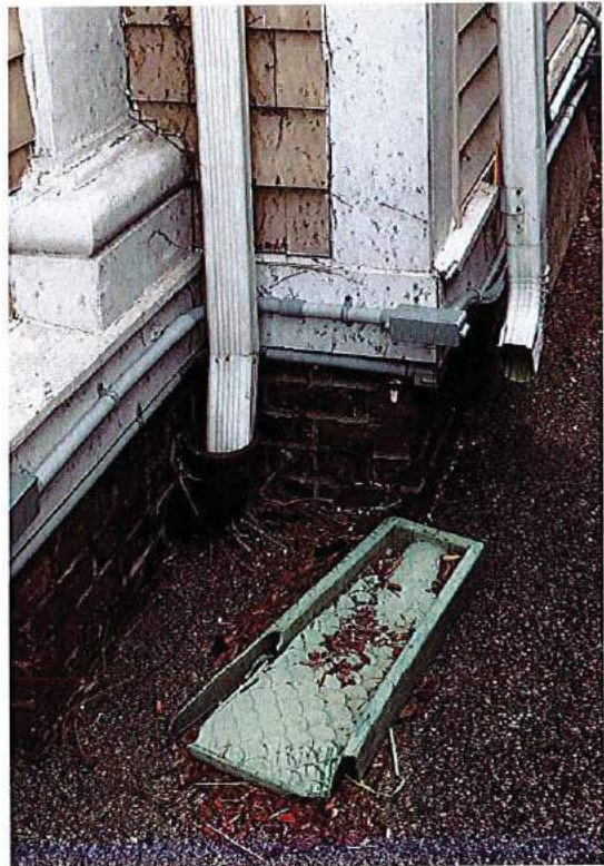
2 Downspouts at the southwest corner
