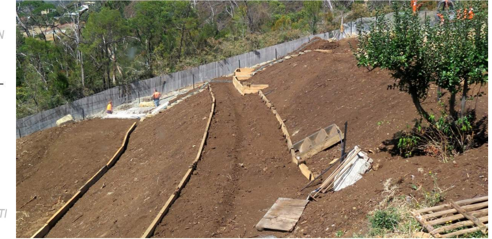
Prepare the slope to receive plants
