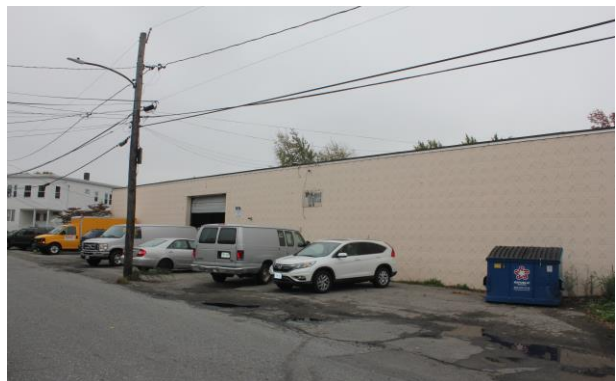
Street view of Murdock Street
