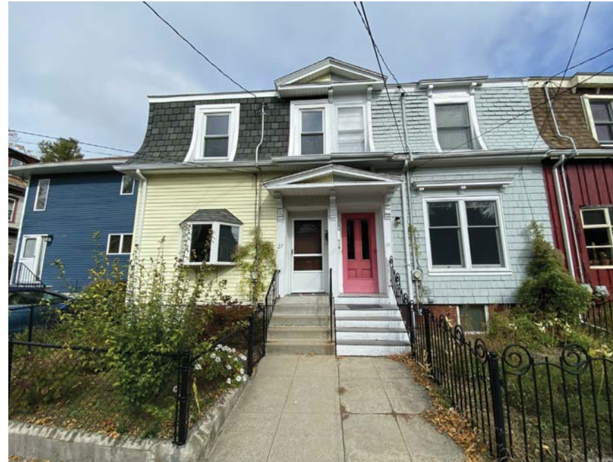
SCOPE OF WORK: SELECTIVE INTERIOR RENOVATION OF EXISTING SINGLE FAMILY DWELLING, BASEMENT STRUCTURAL REPAIRS, REBUILD EXISTING REAR ENTRY MUD ROOM AREA, ADD SECOND FLOOR REAR ADDITION ABOVE EXISTING KITCHEN WING. NO CHANGE TO BUILDING FOOTPRINT.
