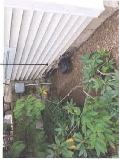
Repair and adjust existing irrigation system
