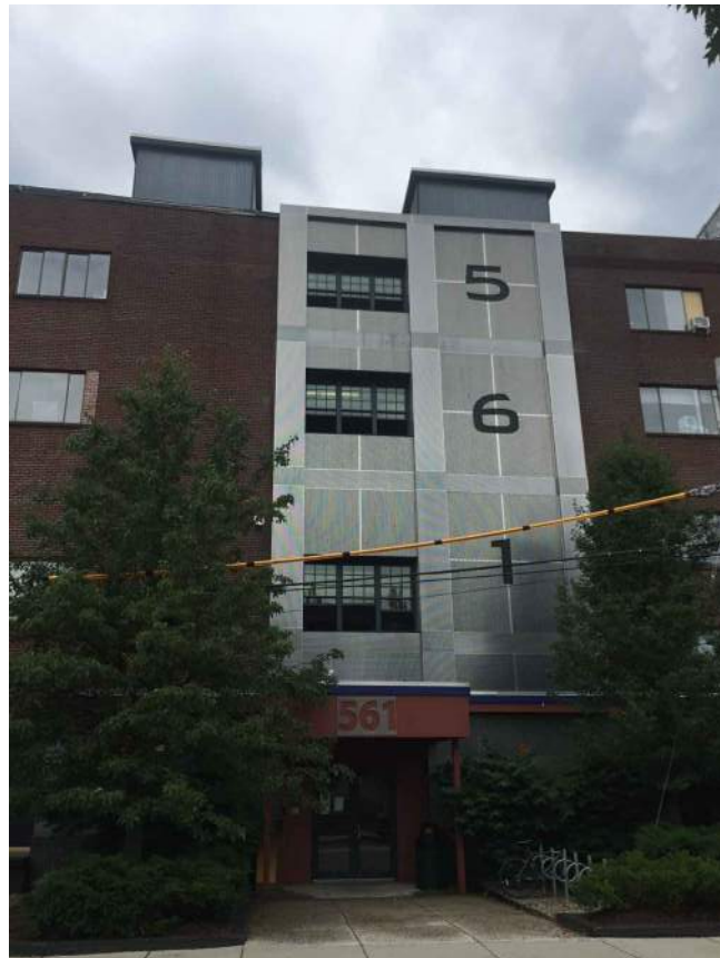
3. EXISTING MAIN ENTRANCE
