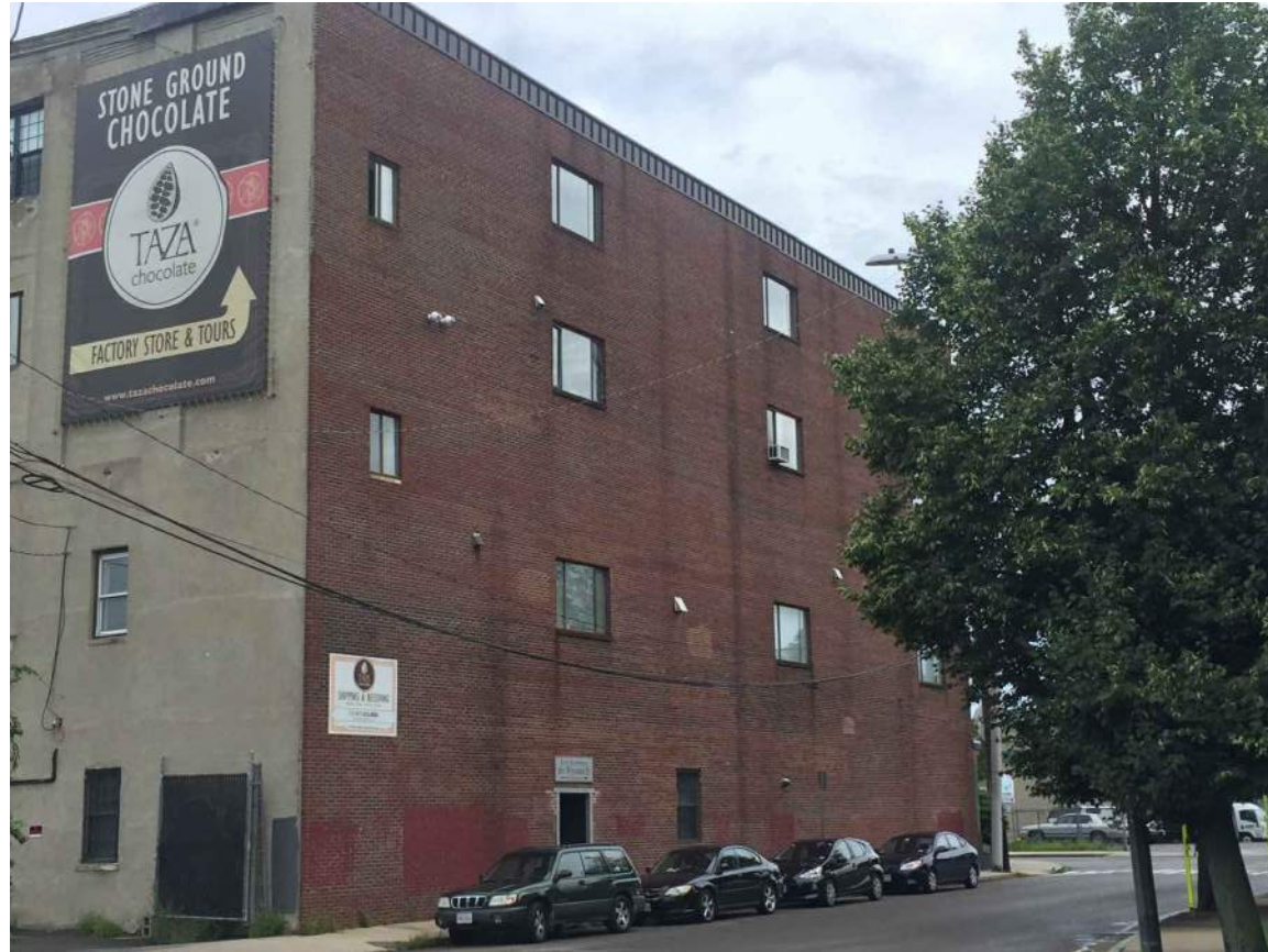
5. EXISTING SOUTH/EAST CORNER
