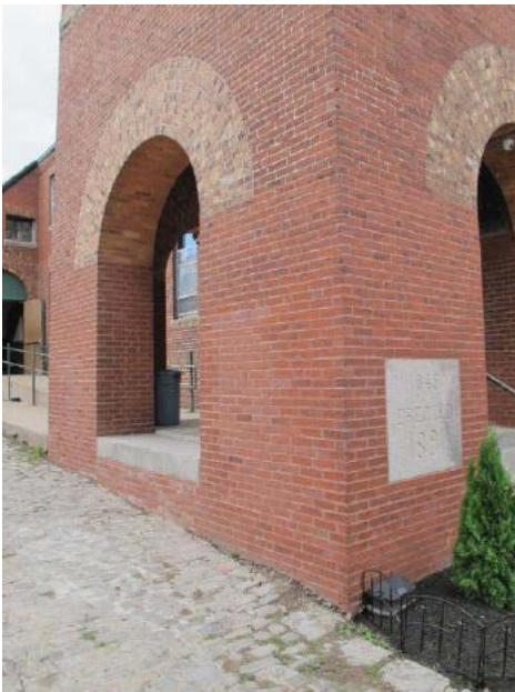
Fig. 1 - Southeast tower, patched and repointed
