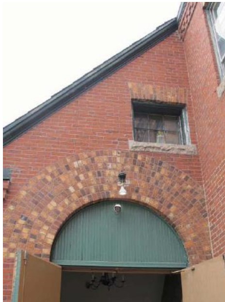
Fig 2 - Entrance following repair of stepped crack
