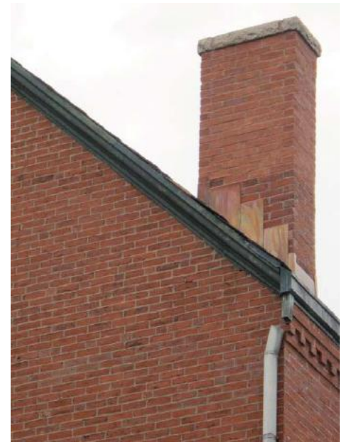
Fig. 3 - Northeast chimney following rebuilding
