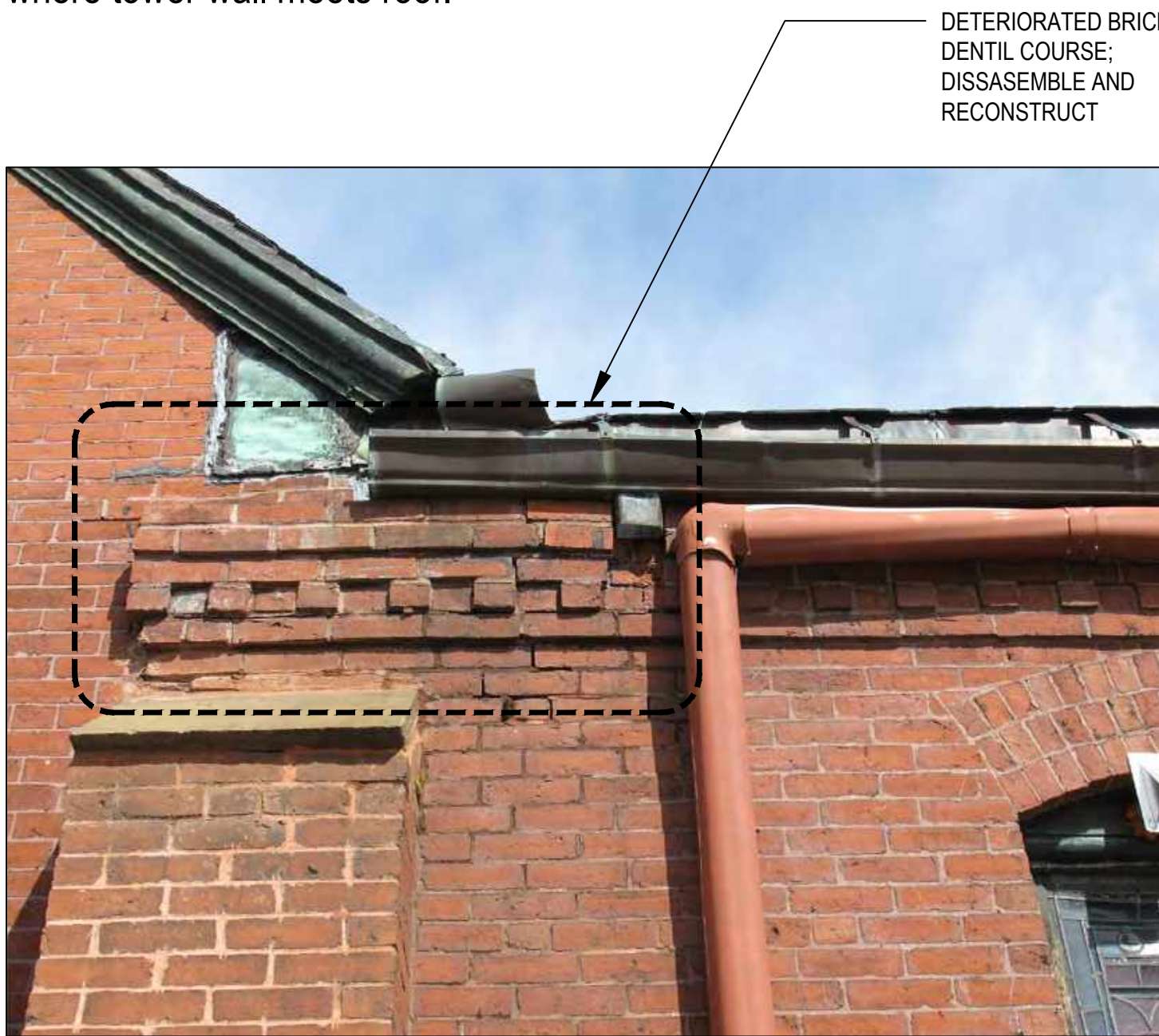
3 4.1 SOUTH ELEVATION - BRICK DENTIL DETERIORATION Scale: 1/8"=1'-0" @ 24 X 36 PRINT
