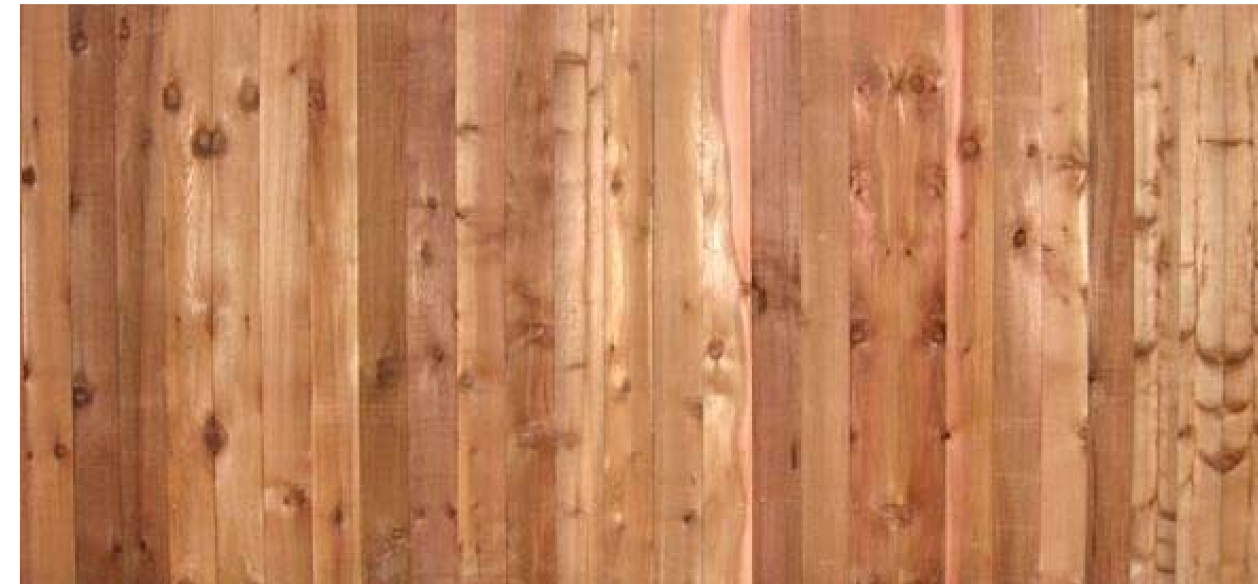
EXTERIOR WALL COVERING - PT CEDAR BOARDS
