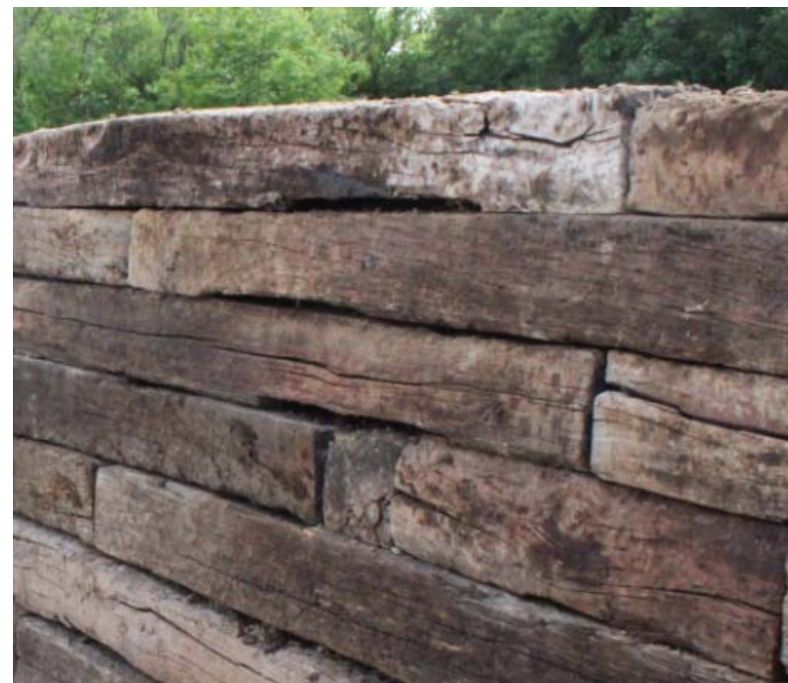
REAR YARD RETAINING WALL - SALVAGED RAILROAD TIES STACKED AND SPIKED TOGETHER
