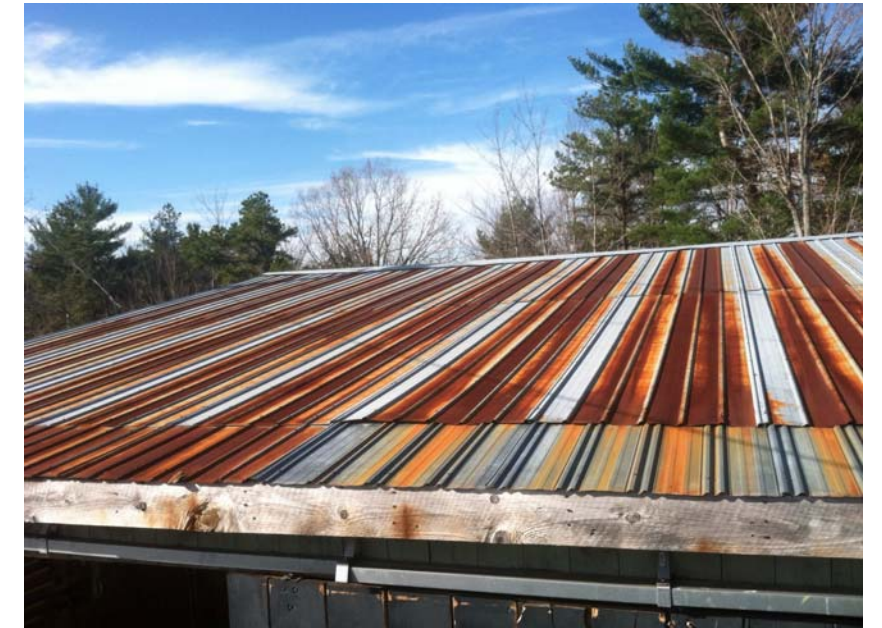
RECLAIMED CORRUGATED METAL ROOFING FOR CANOPY
