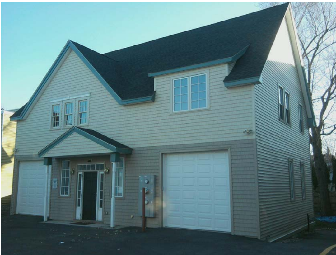
Existing Two Unit Commercial Building at the Rear of the Property
