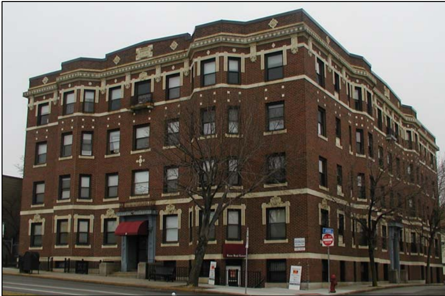
331-333 Broadway, Princeton Apartment Building
