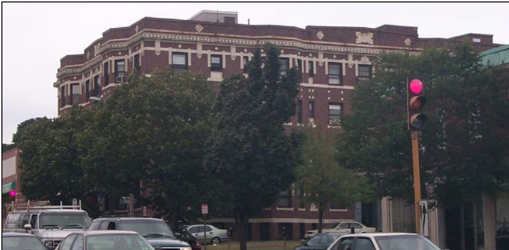
331-333 Broadway: View from Langmaid Avenue to illustrate minimal visibility of three rooftop penthouses and their wireless telecommunications equipment.
