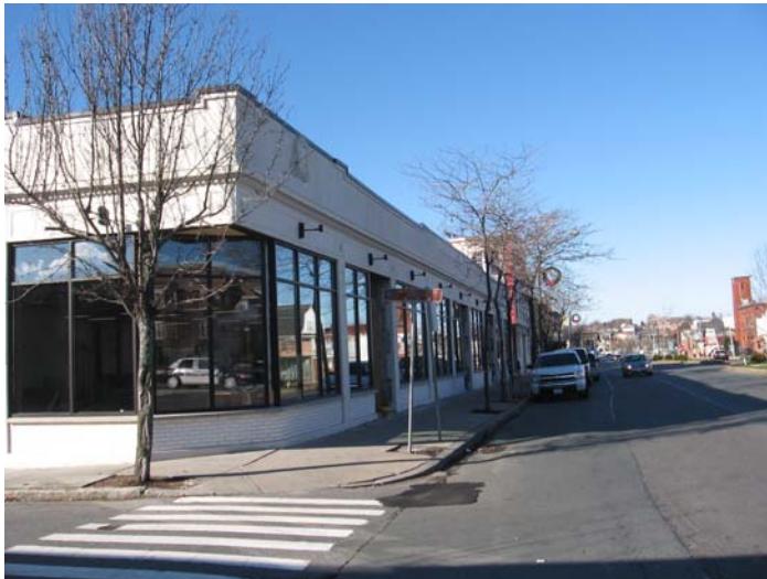
130 Broadway – (top left) Current conditions after renovations
