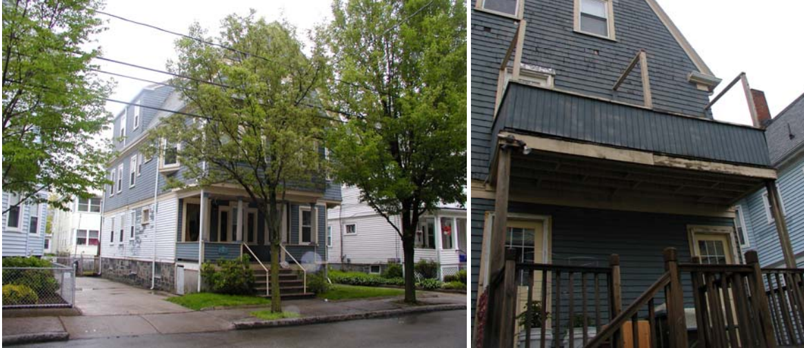
61 Bromfield: front of house (below), existing deck (right)
