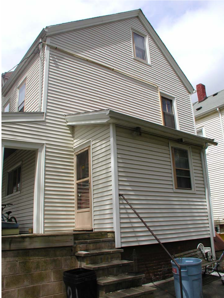
Existing Rear of Structure
