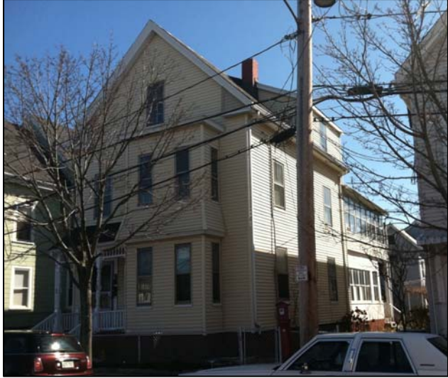
Left: 11 Church Street, front (West) and side (South) elevations
