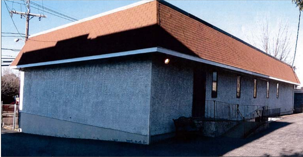
11-13 North Street: Rear and right side façades
