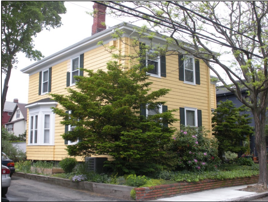
Existing conditions, 142 Orchard St.
