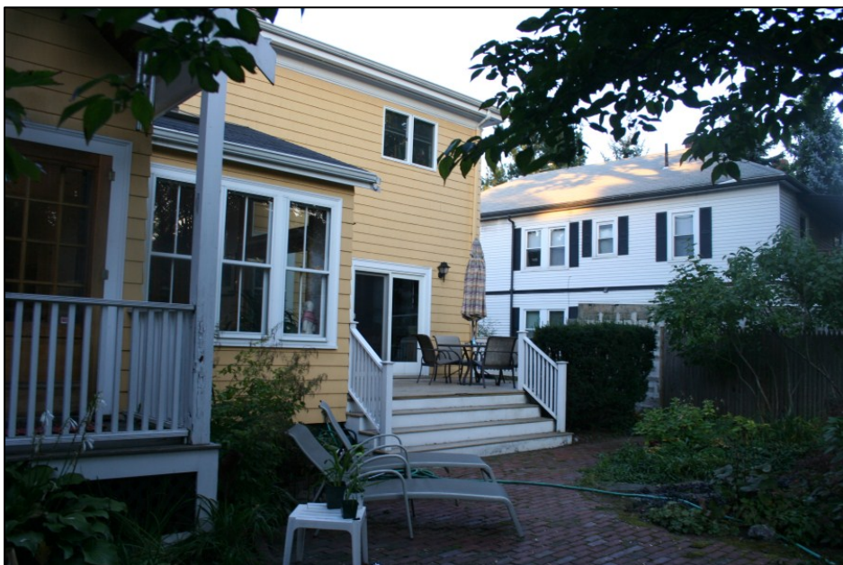
Rear façade, including existing deck and rear porch
