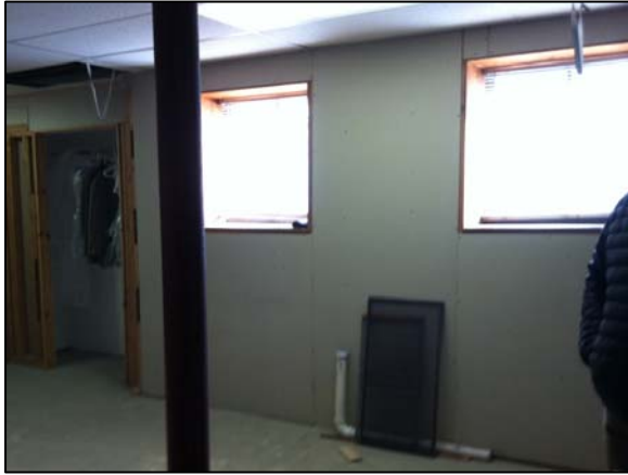
Left: Basement windows for Unit 1
