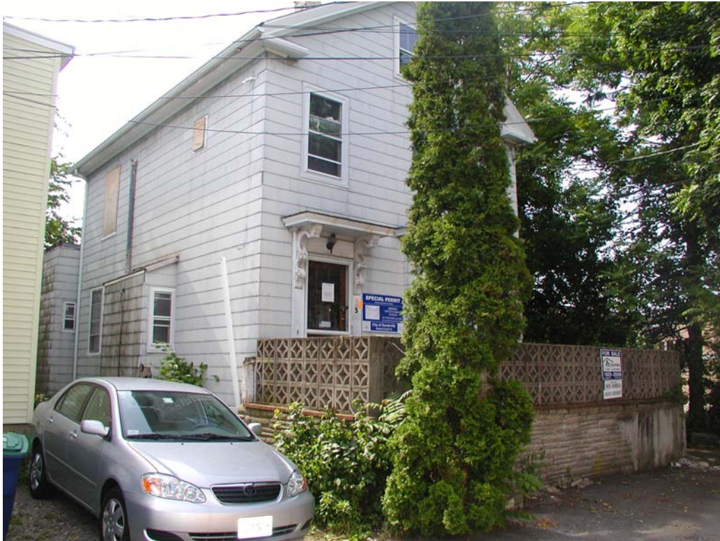
Existing Conditions, Looking from Tower Court, Highlighting the North Side
