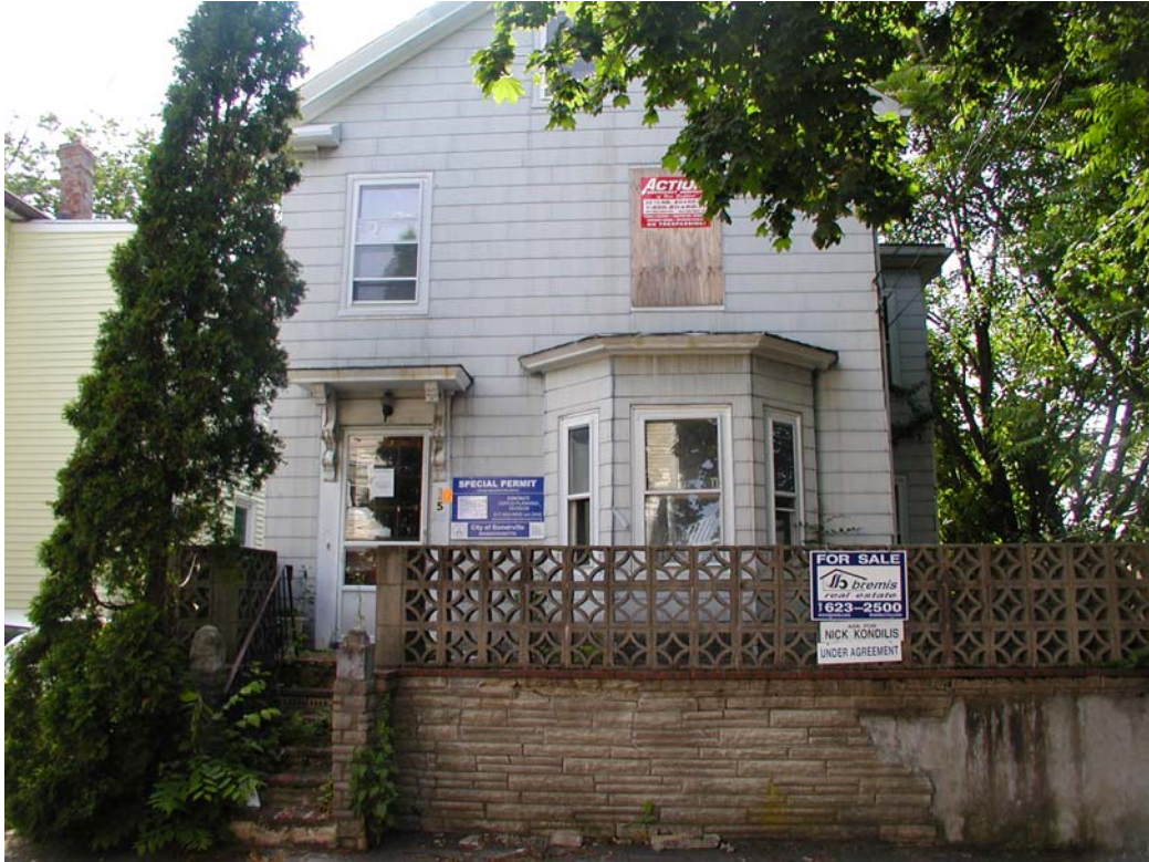
Existing Conditions, Looking from Tower Court, West Side of Existing Structure
