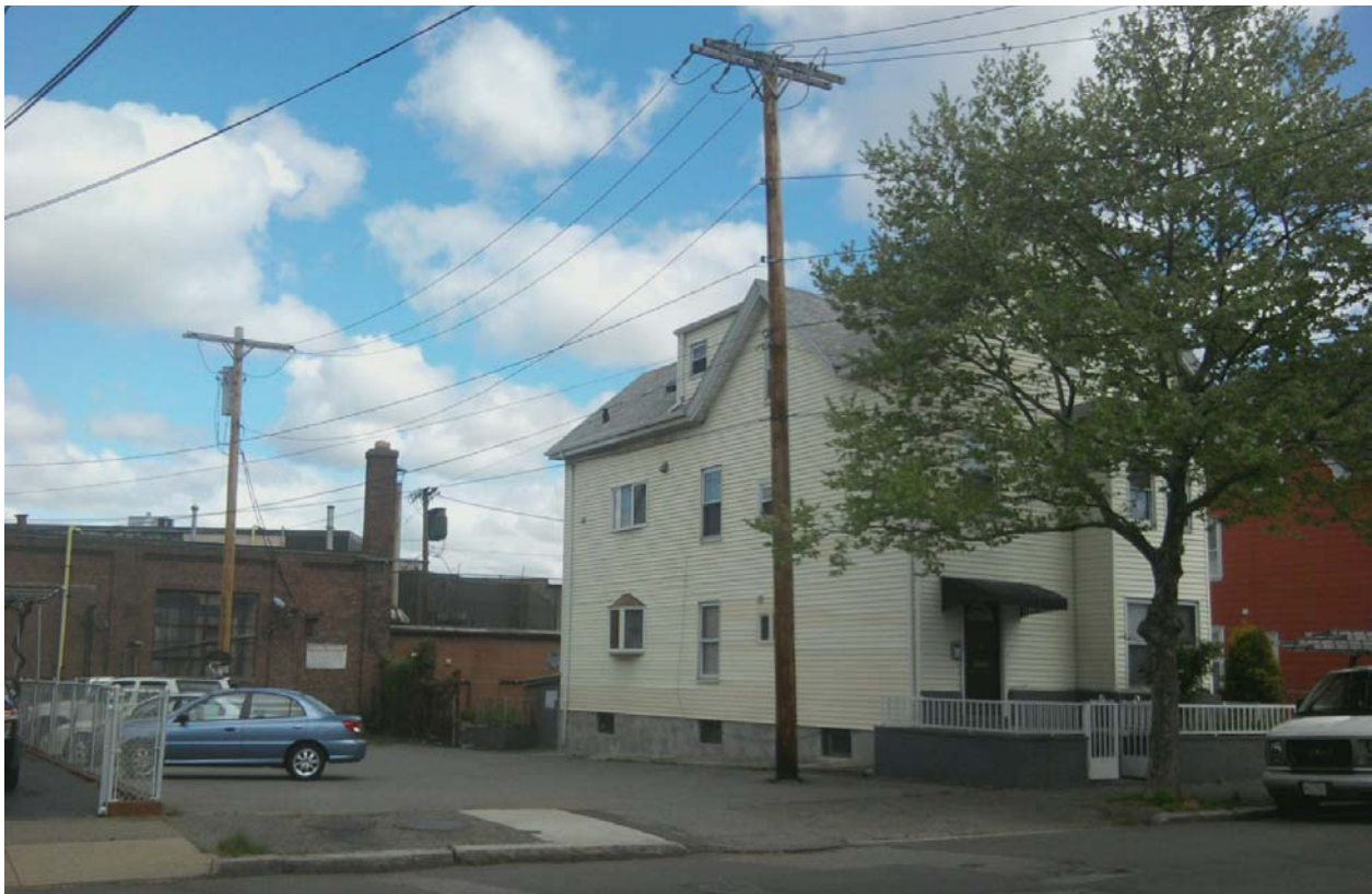
Existing Structure and Parking at 331 Washington Street
